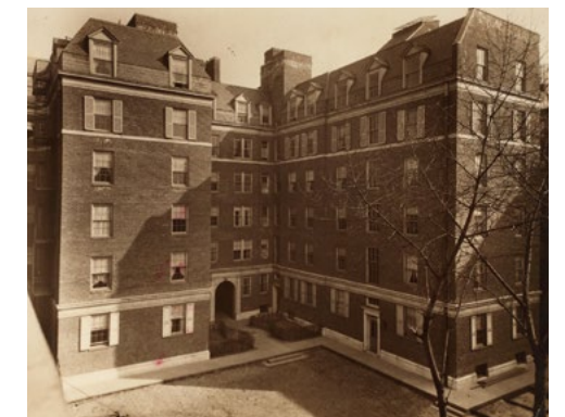
View of rear of Union Settlement Apartments in 1929. Photo from NYPL Digital Collection.
