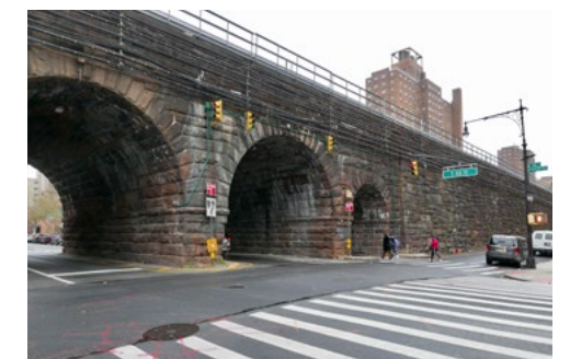
Top: The beginning of the steel viaduct at E. 111th St; bottom: the stone viaduct at E. 106th St. Nov. 2021
