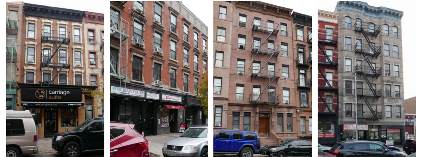
From left to right: 172 E. 104th St, one in a row of five tenements built in 1879. The four-bay facade is often a telltale detail of a tenement; 155 E. 103rd St is one in a now-combined row of five neo-Grec-style tenements called “The Sonyea,” built in 1880 and which fire insurance maps reveal have generously sized interior lightwells by the standards of the day; 169 E. 102nd St, one in a row of six tenements designed by architect John Hauser in 1892 with two units per floor and a bit of refinement in facade dressing; 1791 Lexington Ave, built in 1904 is an example of a new-law tenement on a lot less than 40 feet wide.
