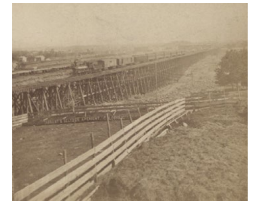
A stereograph of the New York & Harlem Railroad in 1870 showing the temporary timber trestle over the Harlem Flats. From New York Public Library Digital Collection.
