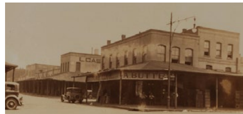
Top: Nov. 2021; bottom: the buildings as two of them (in the far distance) appeared in 1929 (NYPL Digital Collection)
