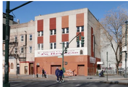
Today a church, the former Park Palace at 1332 Fifth Avenue is located immediately beyond the boundaries of this survey area. It is a significant cultural landmark worthy of preservation.
