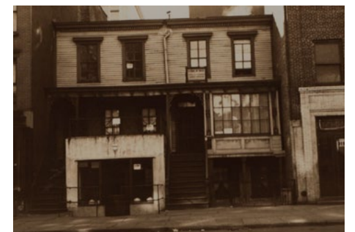
Top: 2034 Third Ave as seen from 112th Street in 1934. Middle: The same building as seen from Third Ave in 2021. Bottom: 304-306 E. 109th St in 1934, no longer extant. Archival photos by P.L. Spurr, NYPL Digital Collection.
